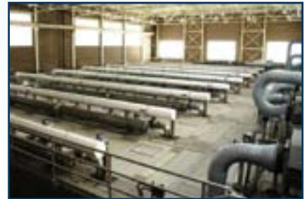
View of the housing deck for the membrane filters and vacuum system
