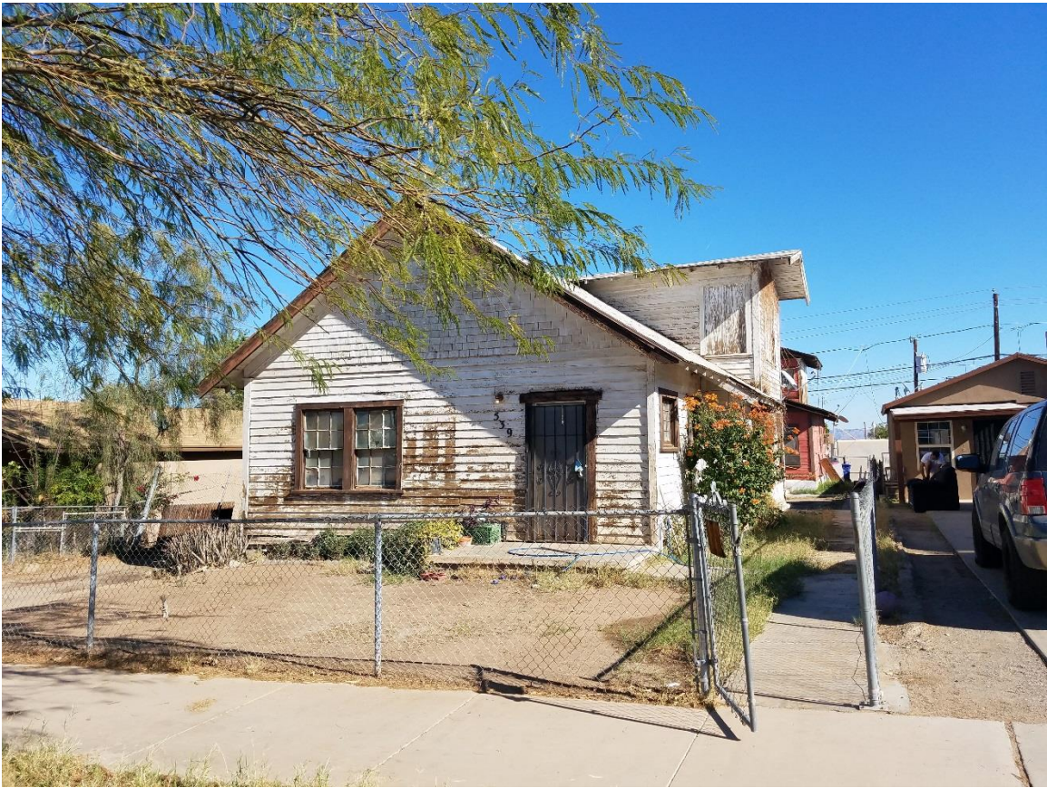
View of 539 S. 2 nd Avenue, facing east
